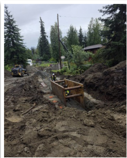
Photo caption: HC trench box in Fairbanks, Alaska.
